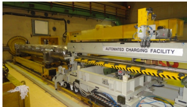
Fig 3A: Automated Charging Facility at P3A
