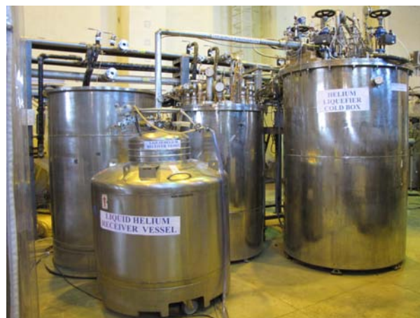
Figure 2. Modified Claude cycle based helium liquefaction/refrigeration system (4.5 K) [1].
