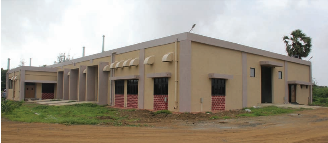
Fig. 1: Photograph of Electrical Block (132)
