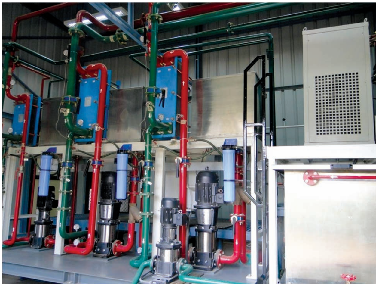
Fig. 5: Cooling Water System for Melter and Generators
