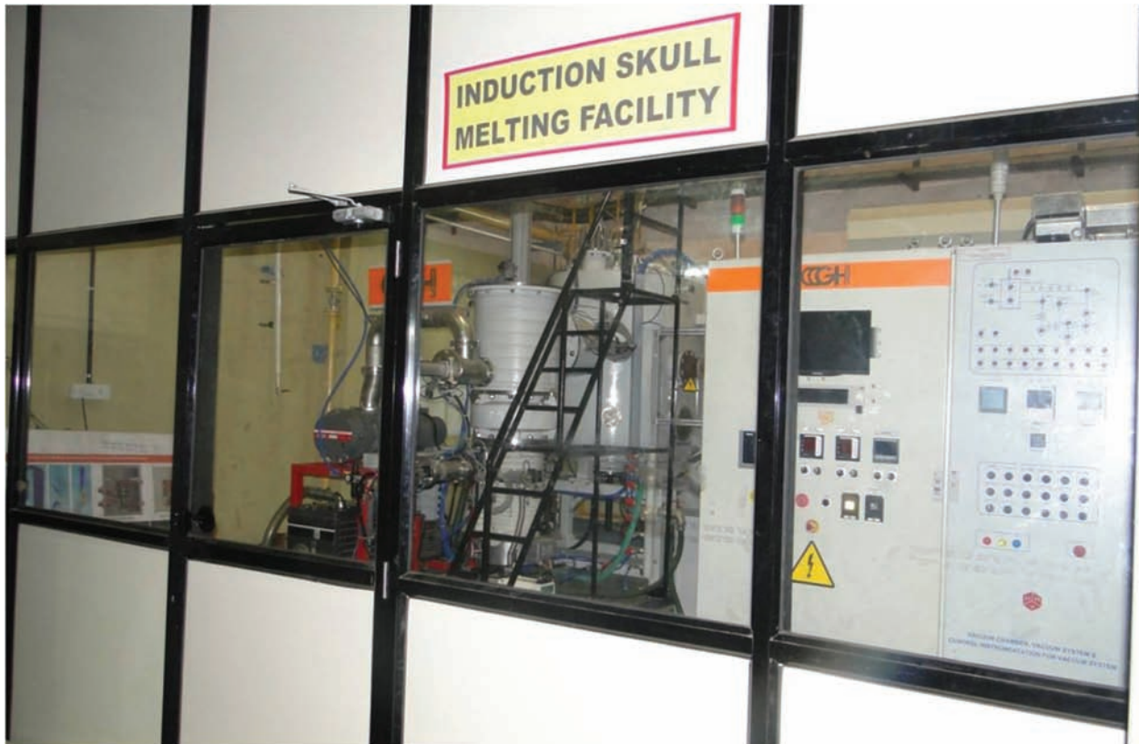
Fig. 2: Induction skull melting facility in BARC
