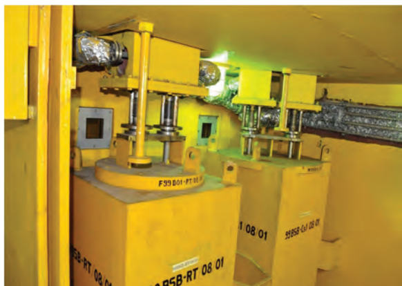
Fig. 4 : Self-shielded ion exchange columns in MS cubicle
