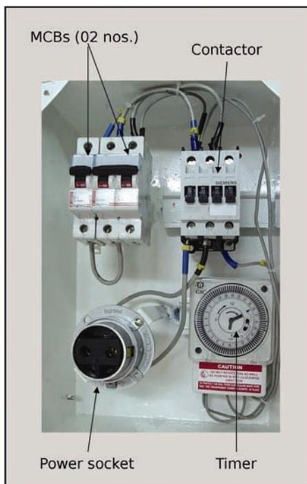
Fig. 3: Timer Control Device
