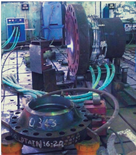
Fig. 5: 600 NB Elbow with Induction heating system
