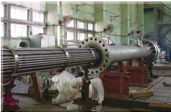
Fig. 11 : One-by-one assembly of the shells on the 11.5 meter long Tube-Bundle
