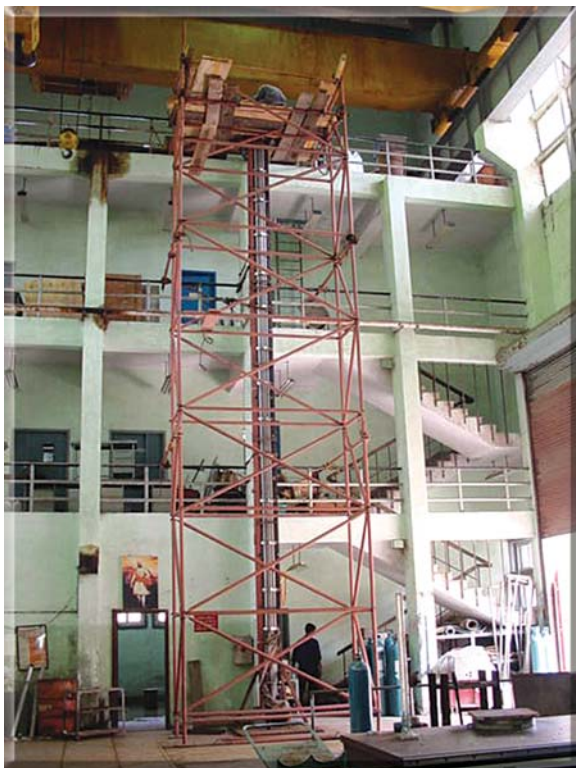
Fig. 9 : Vertical set up for Tube Bundle for welding of tube-to-tube sheet
