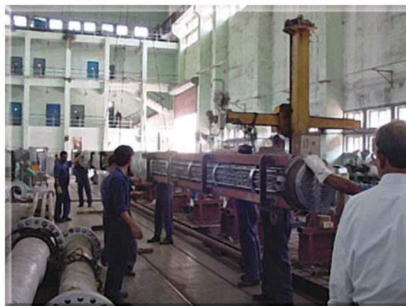
Fig. 8 : Tube Bundle Assembly being lifted in fixture
