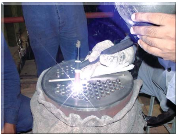
Fig. 10 : Welding of Incoloy-800 Tubes to Tube sheet, in 1G position
