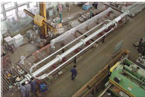
Fig. 12 : Final assembly of Steam Generator
