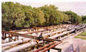
Fig. 11 : Wet test loop at IOC, Faridabad
