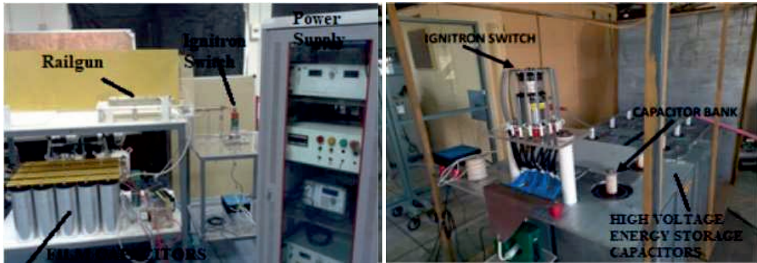
Figure 35.3. Photograph of capacitor bank (a). 2 mF, 20 kJ and (b). 1.78 mF, 200 kJ.
