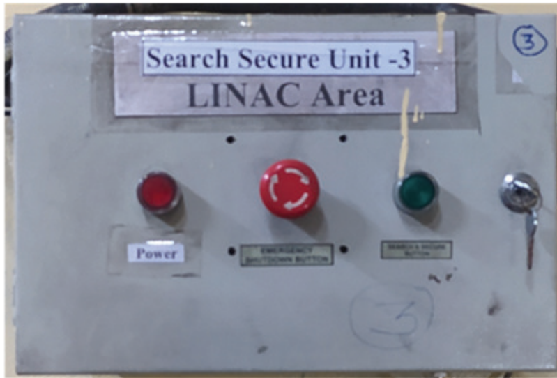
Figure 12.2: Search secure panel in 10 MeV cell area.
