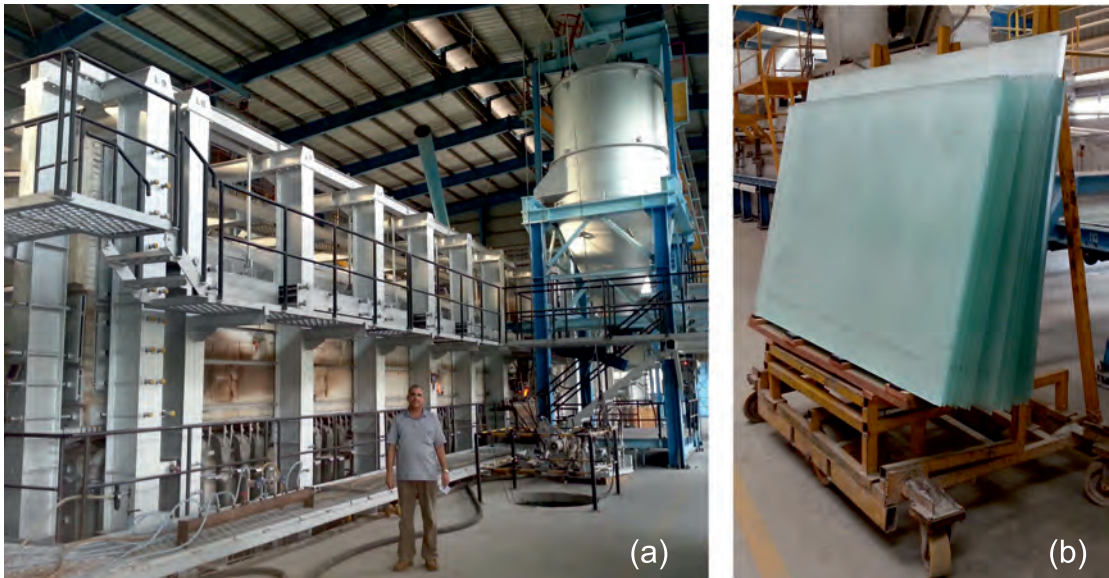
Figure 6: (a) Photograph of a furnace and (b) Produced glass sheets
