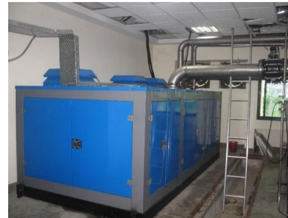
200bar, 660lpm power pack with sound proof enclosure
