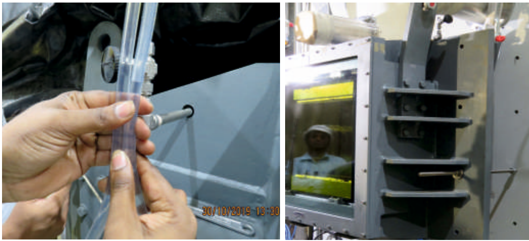
Fig. 3: Installation and Pressure Testing of RSW
