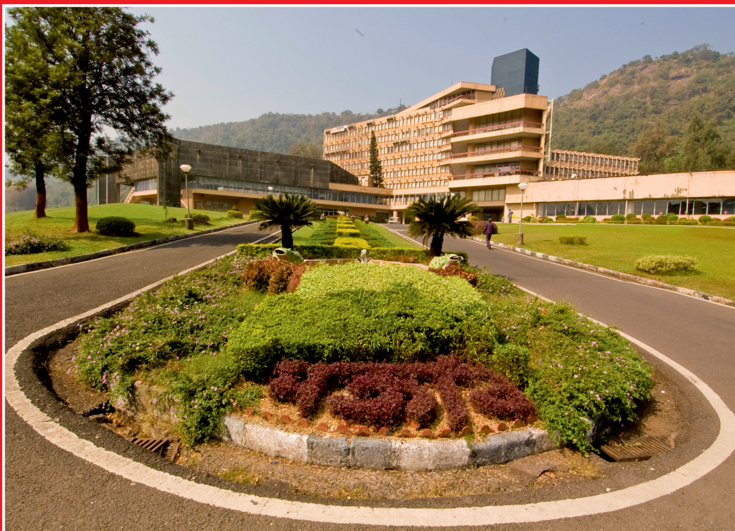
Central Complex BARC
