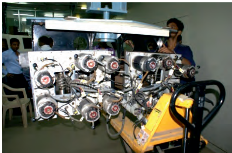
Disconnection of motor cables
