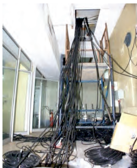
Figure 10. Inactive cabling
