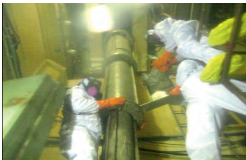
Figure 11. Cable take-up installation inside the hot-cell
