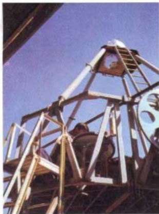
Fig. 4 Alignment work in progress
