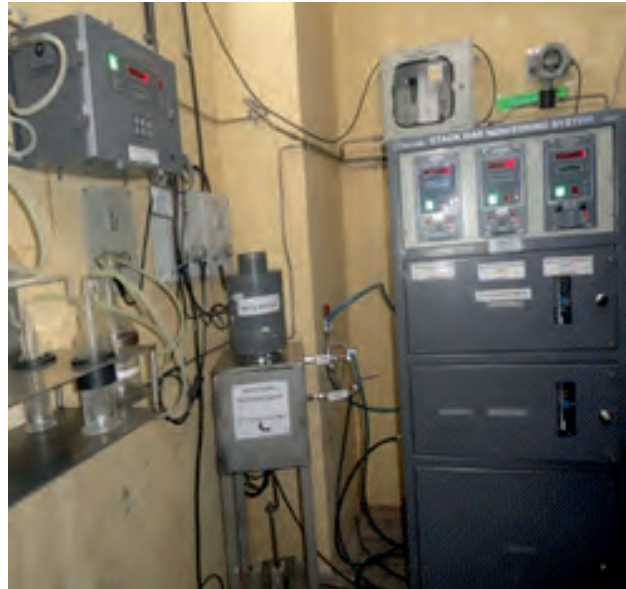
Iodine-129 monitoring system coupled to a stack monitor.
