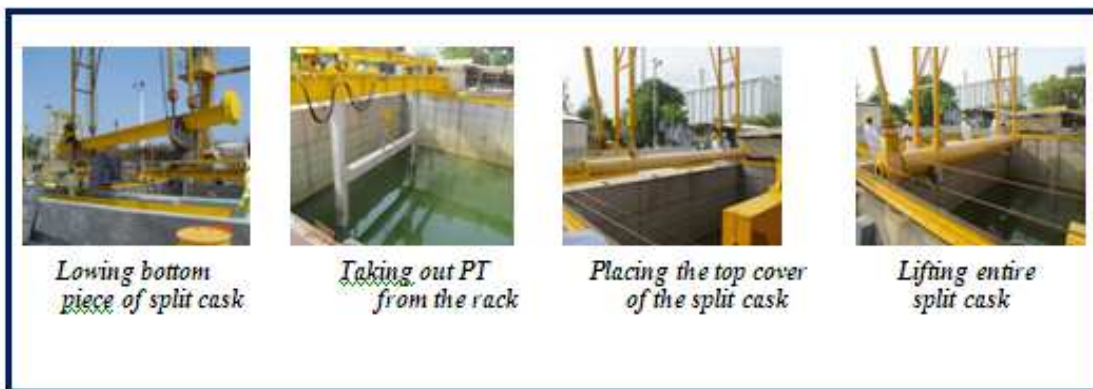
Fig.2: Operation carried out in the storage pool
