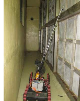
Fig. 7: Trials at HEPA Filter Room, WIP
