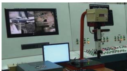
Fig.2: Master Arm of SSM in the Control Room
