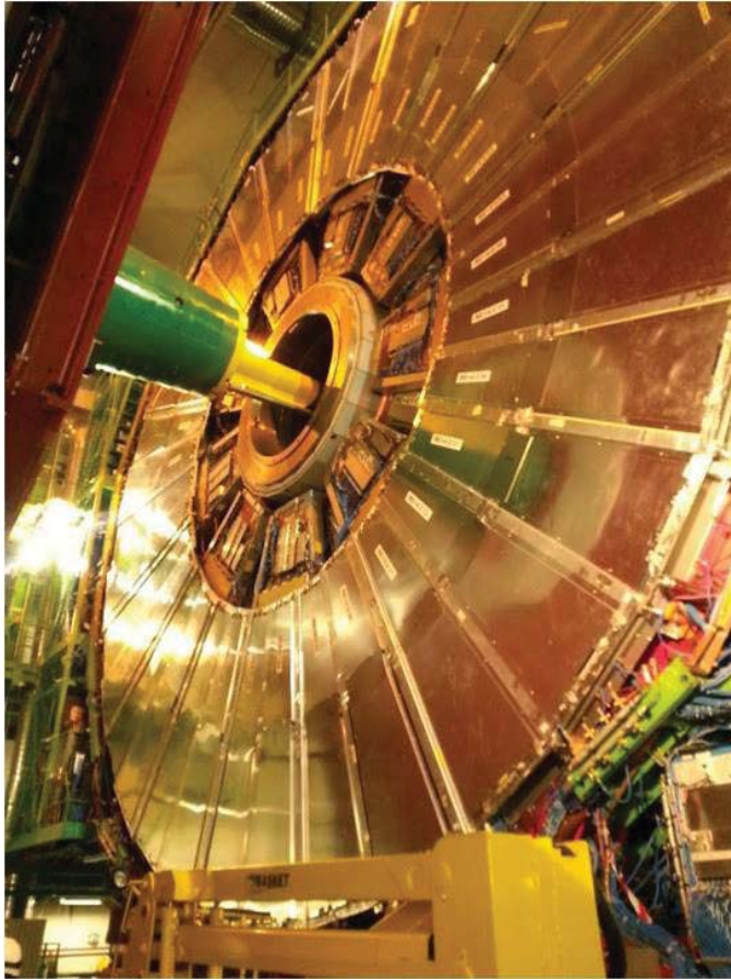
Fig. 2 : The recently installed, positive side of the RE4, 100 metres below the ground, at Point 5 (CMS at the LHC facility) in Cessy, France is approximately 15 metres in diameter, weighing close to 5 tons
