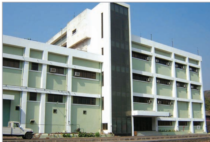
Re-engineered Uranium Metal Plant (RUMP) at South Site, BARC
